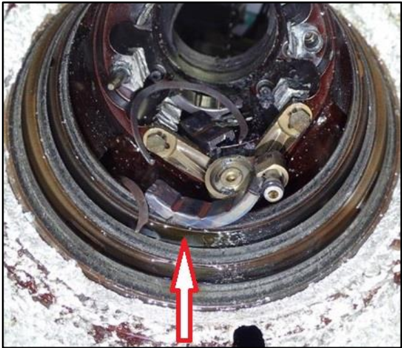
Remains of no. 2 bearing
